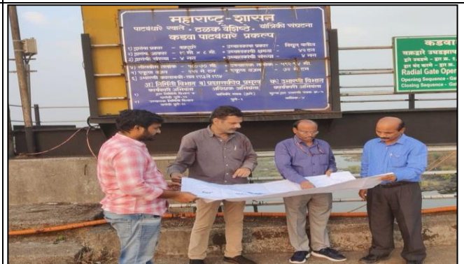
Visit of NWDA officers to Kadwa reservoir outfall site for Damanganga Vaitarna Godavari intra State link project
