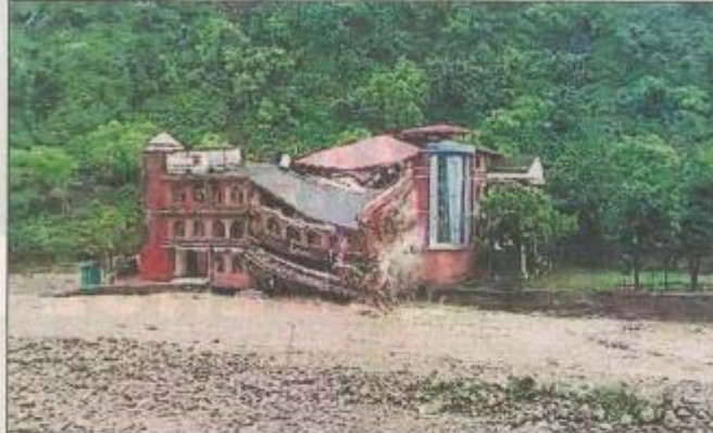
A coaching institute constructed on the riverfront in Rishikesh collapsed amid heavy rainfall (left); while several roads were blocked due to landslides and flashfloods across Uttarakhand on Monday.
